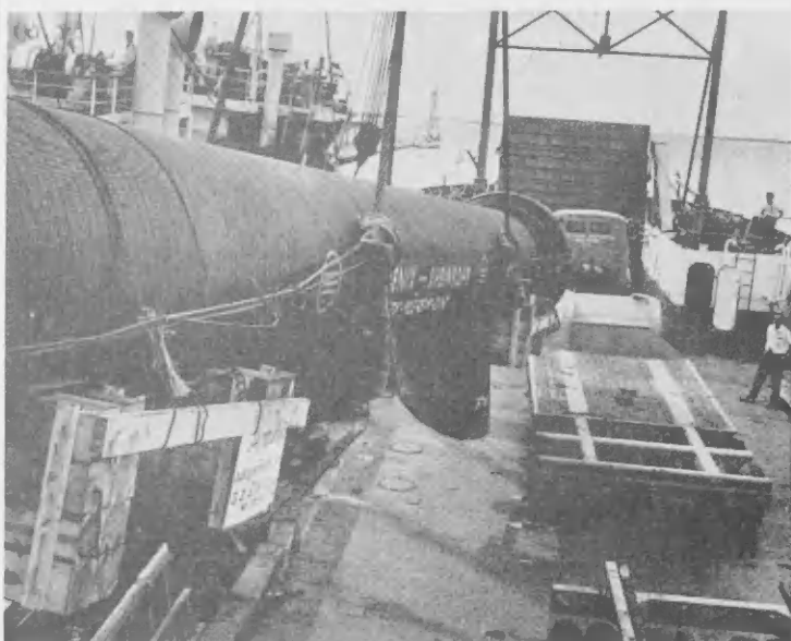
BY MEANS of the Pericles' heavy-duty long-reach boom, the converter is eased onto a special low-boy rig which rests on the deck of the landing craft. The base of the converter is supported on a separate set of wheels.
